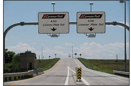
*All-electronic toll collection (AET/AETC) is similar to the EZ Pass system in New York, except that it is typically higher speed and includes cameras for obtaining license plates identification as a secondary collection method for non-EZ Pass holders. © 3M Aylesbury/Denver, CO*
